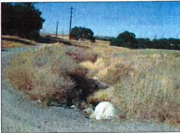
PHOTO 3: View to south of culvert located outside of project site, which drains intermittent surface flows onto the site. This ephemeral drainage rapidly dissipates in the field.
